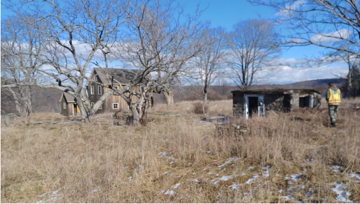
Photo 6: A 1920's house is located in the northern portion of the Project APE, along with several outbuildings. These buildings are associated with the former Toro Hill Farm. View to the northeast.
