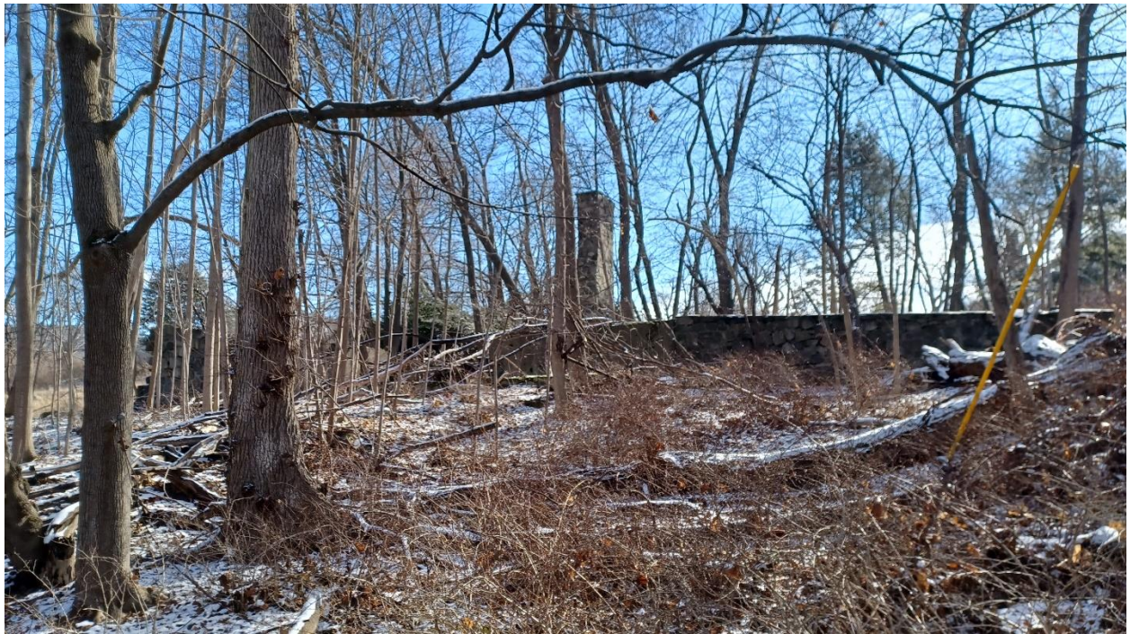
Photo 16: The stone and cement foundation is located to the northwest of the residential structure in the northeastern portion of the Project APE. View to the southwest.
